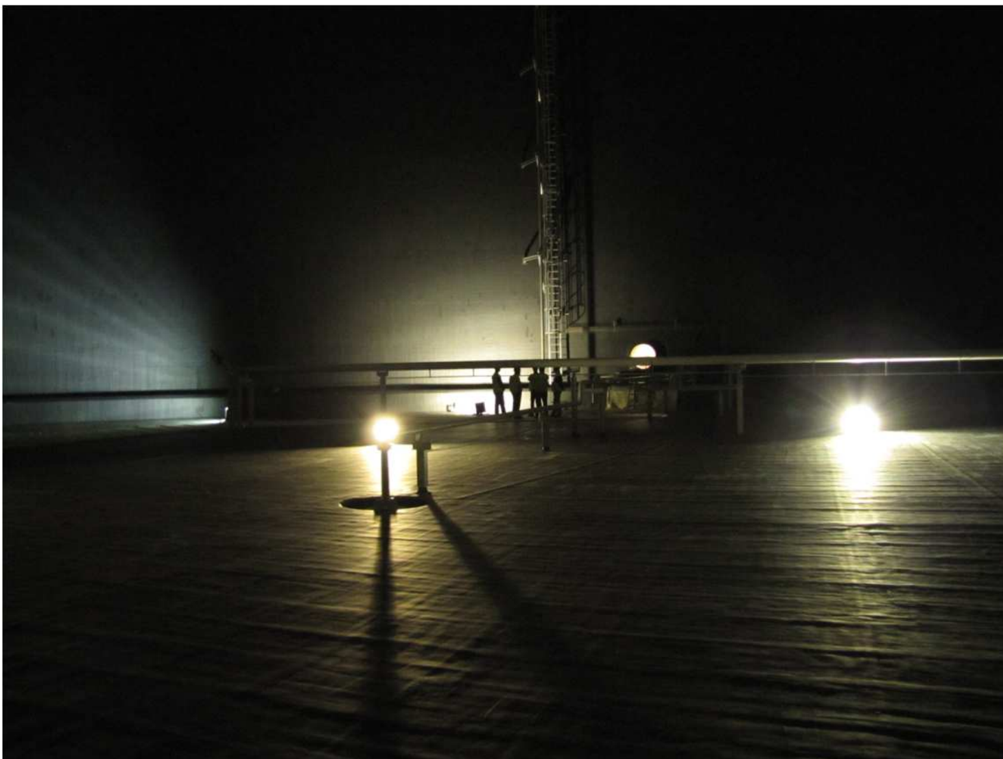
Final check of the tank before filling
