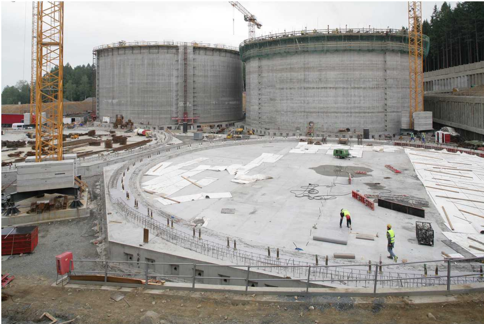
Built of a new tank, Tank foundation (concrete)
