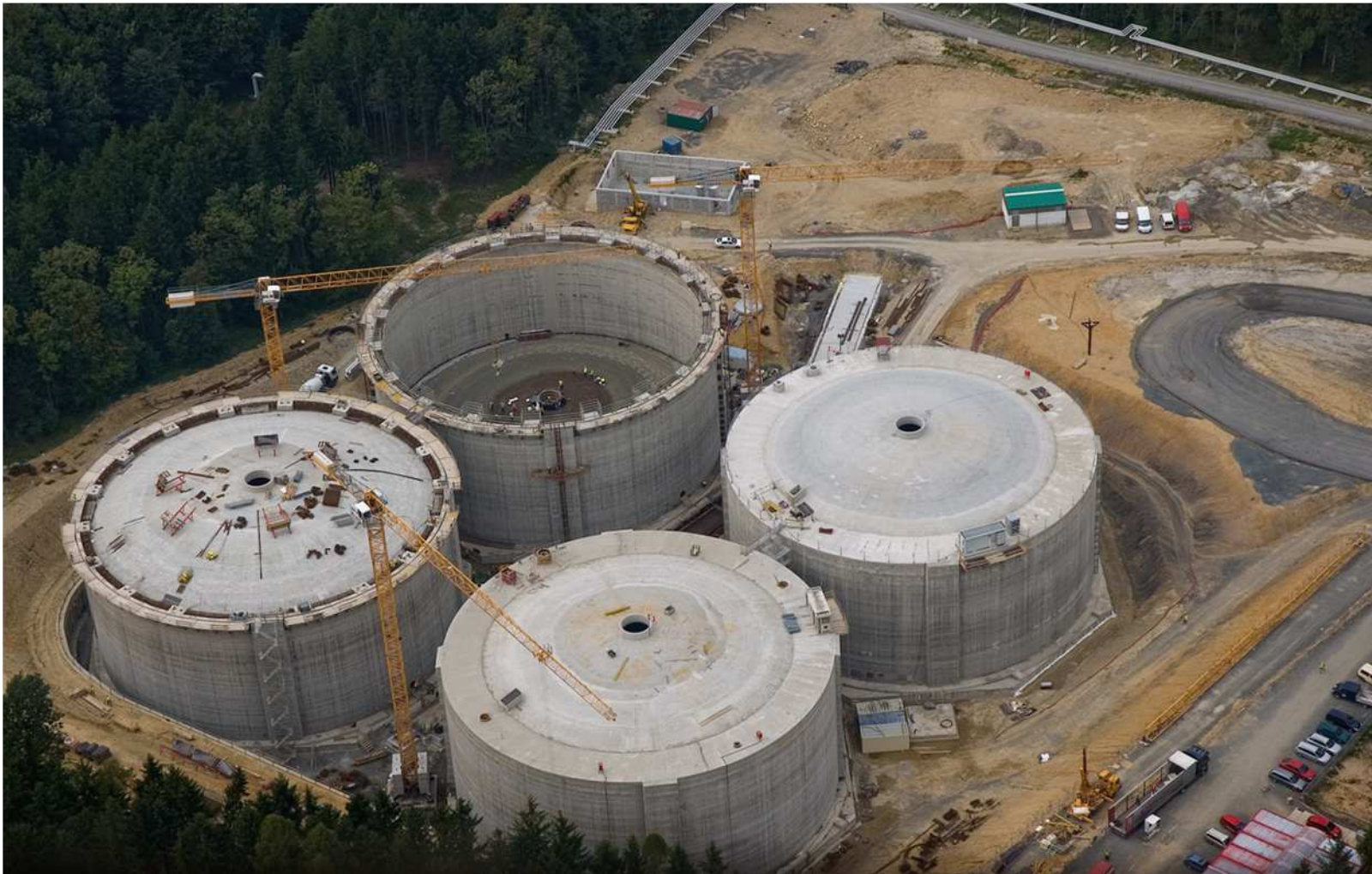
Finished tanks with concrete roofs
